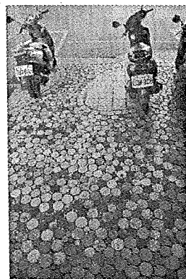
Fig. 19 Disused rock core paving for footpath - 2 (Hualien, Taiwan)
