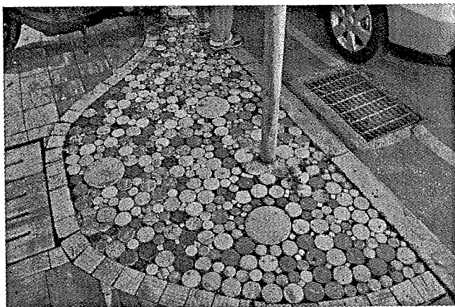
Fig. 18 Disused rock core paving for footpath - 1. (Hualien, Taiwan)
